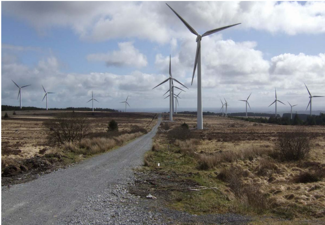
Plate 1. View looking eastwards of unplanted cutover bog in eastern section of site. Hen harriers have been recorded foraging over this area of the wind farm (April 2018).
