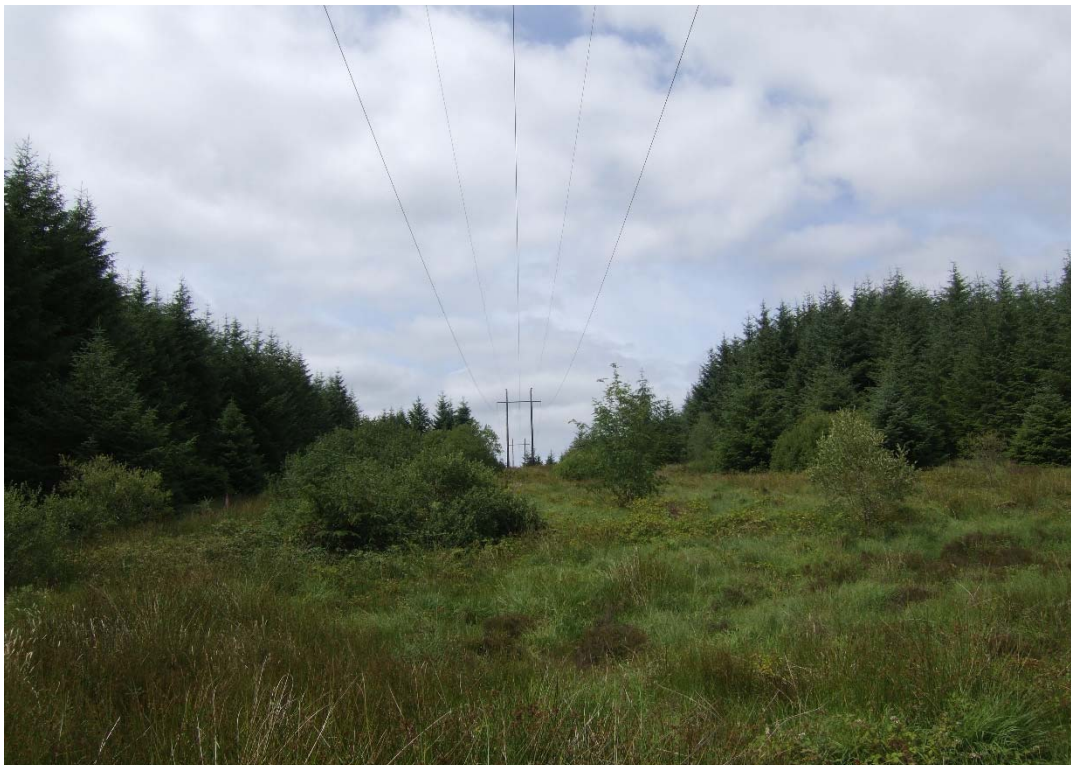
Plate 4. View of overhead line corridor, May 2018. The clearance of conifers has allowed regeneration of bog and heath vegetation, with scrub patches – this provides useful foraging habitat for hen harriers.
